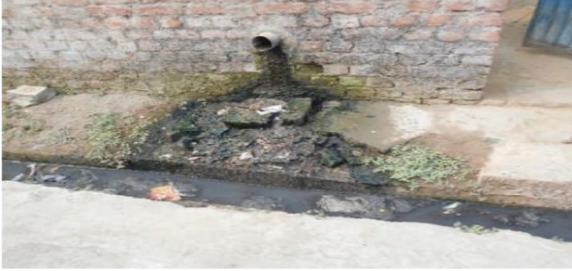
Black water from Septic tank
