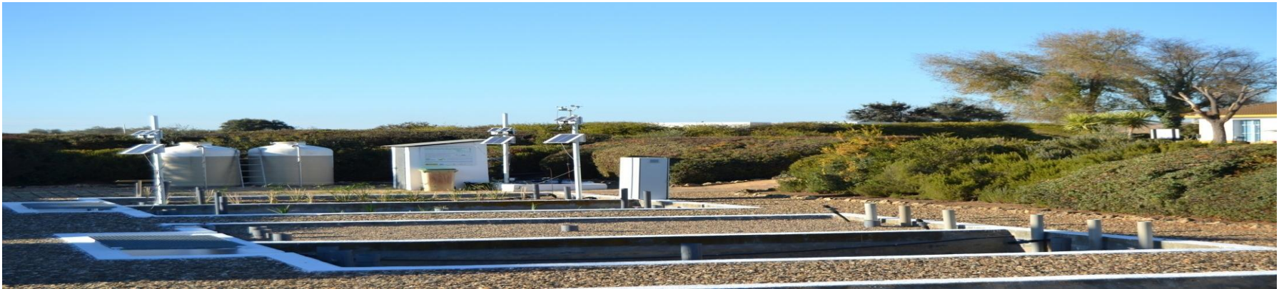
Waste Water Treatment Plant
