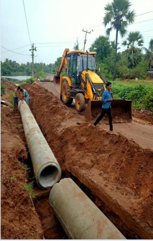
Under ground drain (UGD) under construction and UGD after completion
