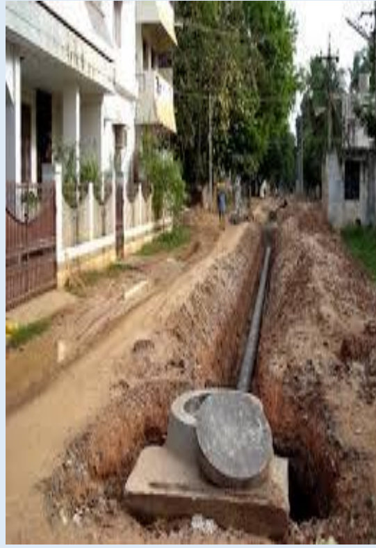
Under ground drain (UGD) under construction and UGD after completion
