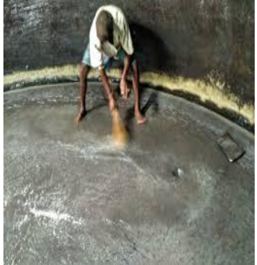
Cleaning and Chlorination
